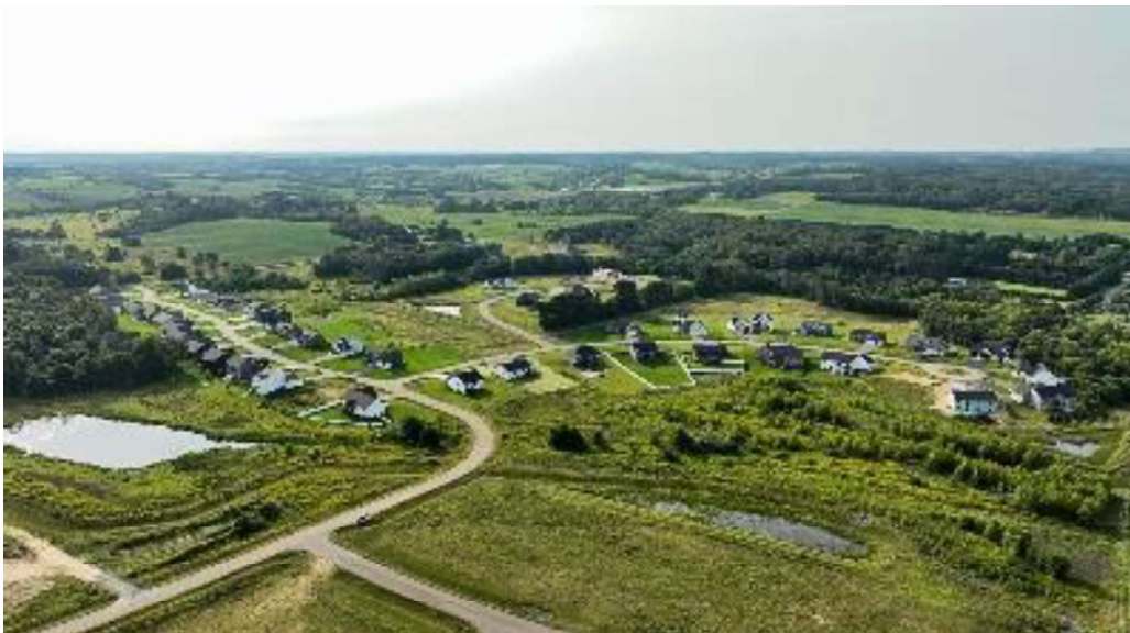
Photo 1: Trilogy subdivision looking south
